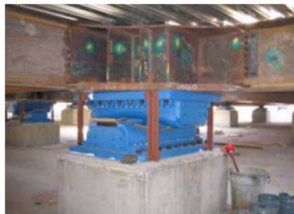
Fig. 14. (a) Three-dimensional view of the uplift-restraining XY-FP isolator (adapted from [79]); (b) Installation of XY-FP tension-capable bearings in LA EOC in California (adapted from [79]).
