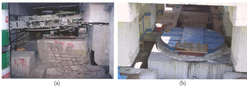
Fig. 8. Bolu Viaduct: (a) view of damaged EDU and loss of beam support; (b) FP bearing positioned on its support, before casting the transversal diaphragm post-tensioned beam.
