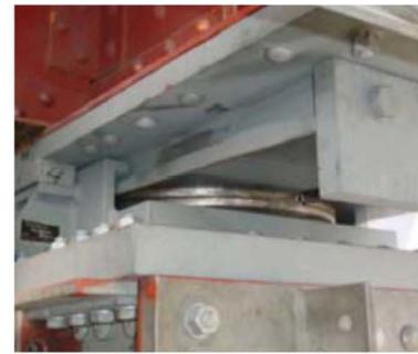
Fig. 12. (a) Section of Teflon Disc Bearing with uplift-restraint devices, and helical spring unit (adapted from [81]); (b) view of unidirectional FP bearing with uplift-restraint installed at the San Francisco approach to the Oakland Bay Bridge (adapted from [79]).
